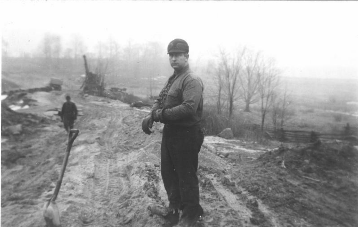
Robert W. Sidley (R.W.) stripping dirt to get to the conglomerate (silica) level in Thompson, OH, 1940's.
