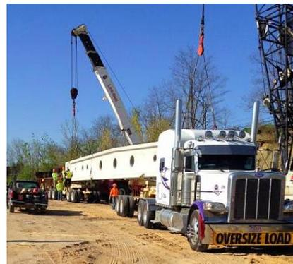
The support beams are for roof structure of Building C, they are made with lightweight concrete and weigh almost 42 tons each and are 84'-8" long x 5'-7-1/4" high. The project includes production and delivery of 54 large beams and 54 smaller beams.
