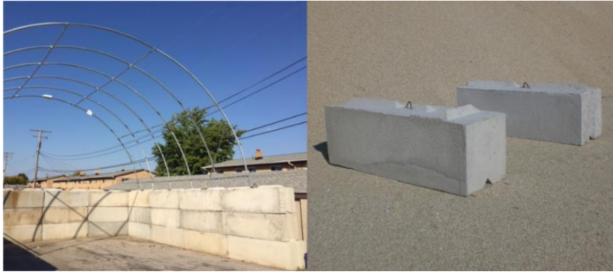
Salt bin storage made from wall blocks.(left) Standard wall blocks.(right)
